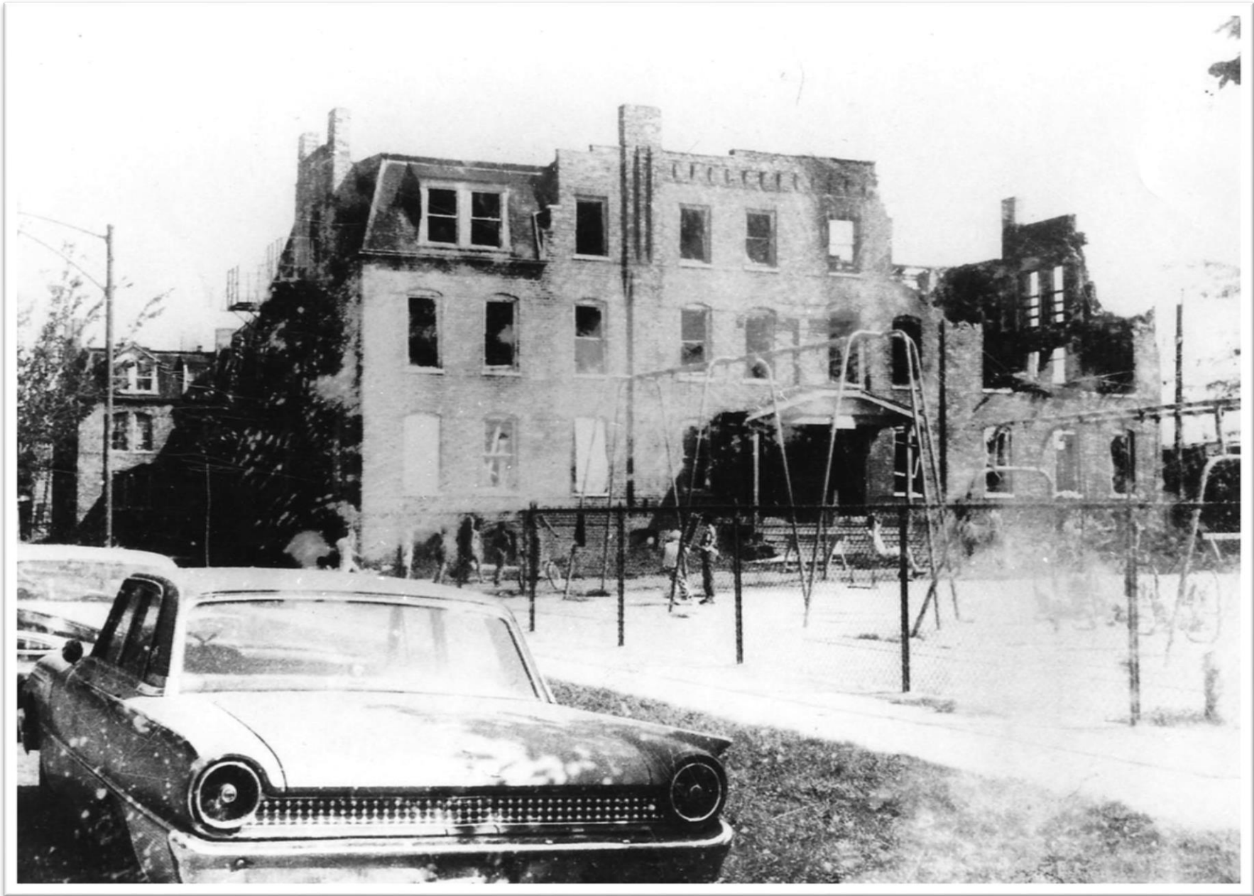
Figure 14. Fire-damaged Tenement "E" circa 1972.
