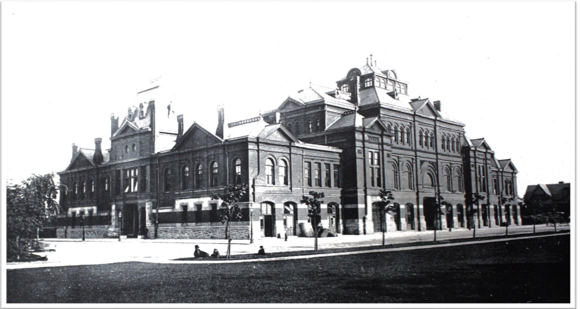
Figure 4. Looking Southeast from the Pullman Depot toward the Arcade and Stables.
