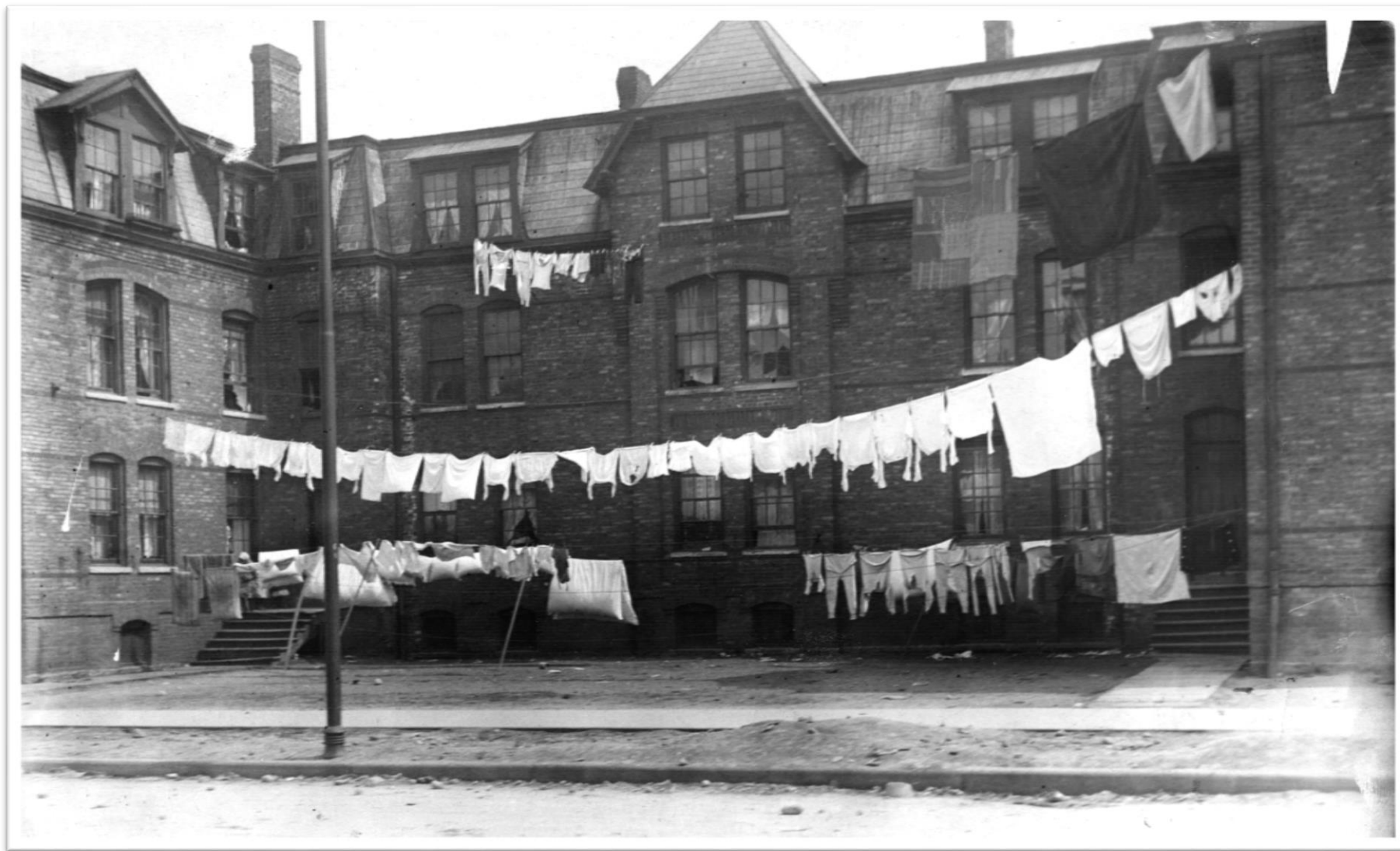
Figure 10. Tenement "D" or "F" as it appeared in 1915. The area within the forecourt was historically not lawn, but instead cinders and slag upon which the children would play and the clothes would drip as they dried. This east facing elevation was duplicated on its west facing elevation.
